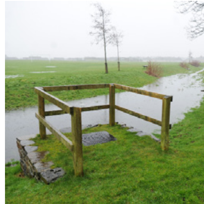
Queen Mary's Walk swale completed summer 2013
