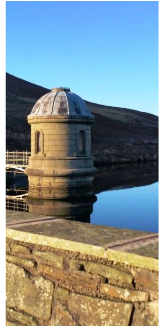
Figure 36 : Upper Lliw Reservoir, Velindre © Welsh Water
