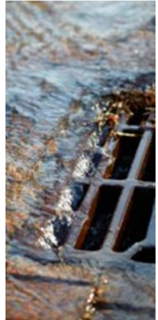
Figure 87 : Drainage © Welsh Water
