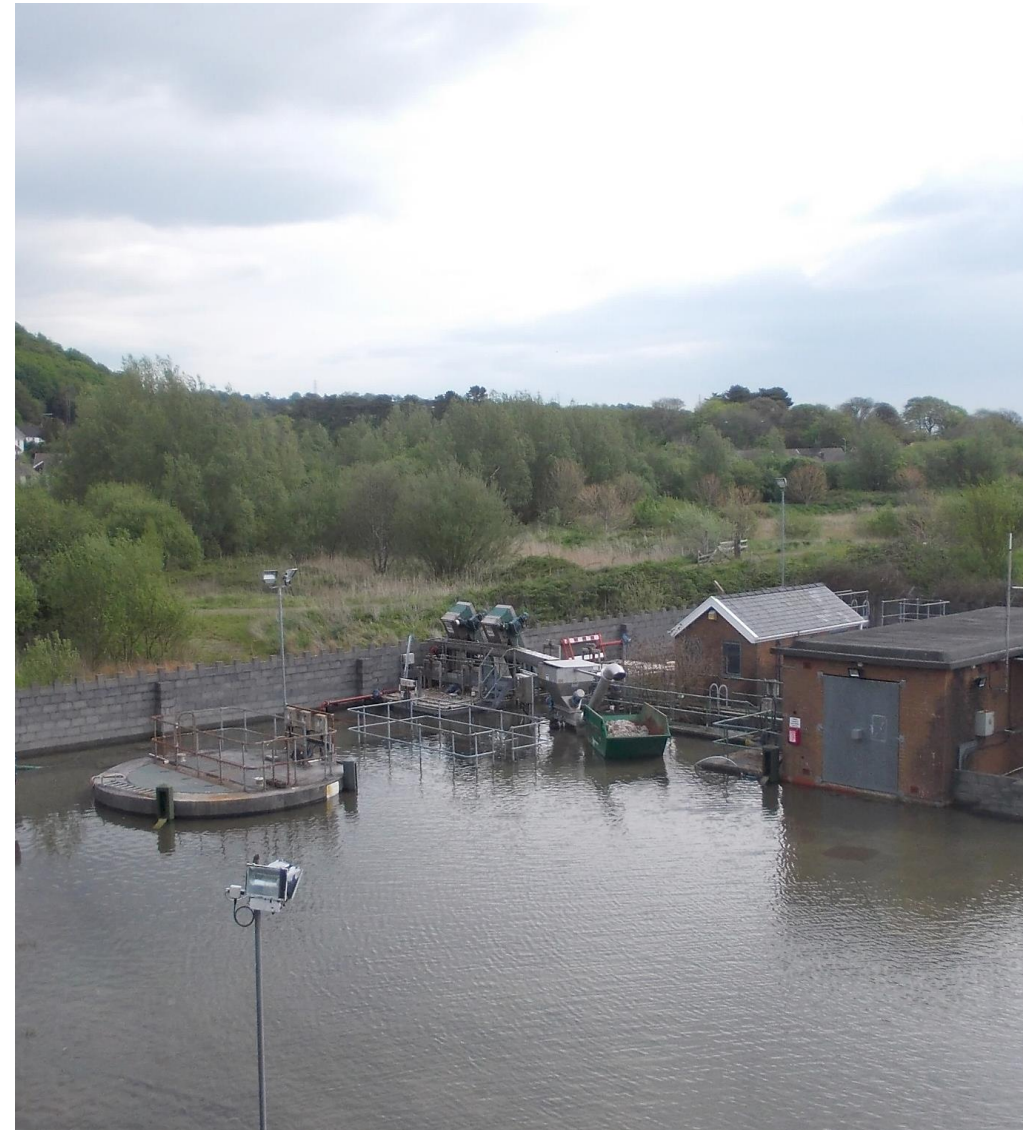
Figure 94 : Pwll Pumping Station experiencing flooding in 2016. © Welsh Water.
