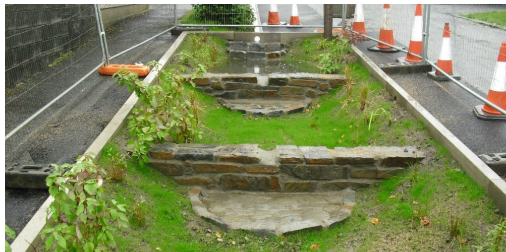
Figure 85 : A rain garden at Queen Mary's Walk, Llanelli. © Arup
