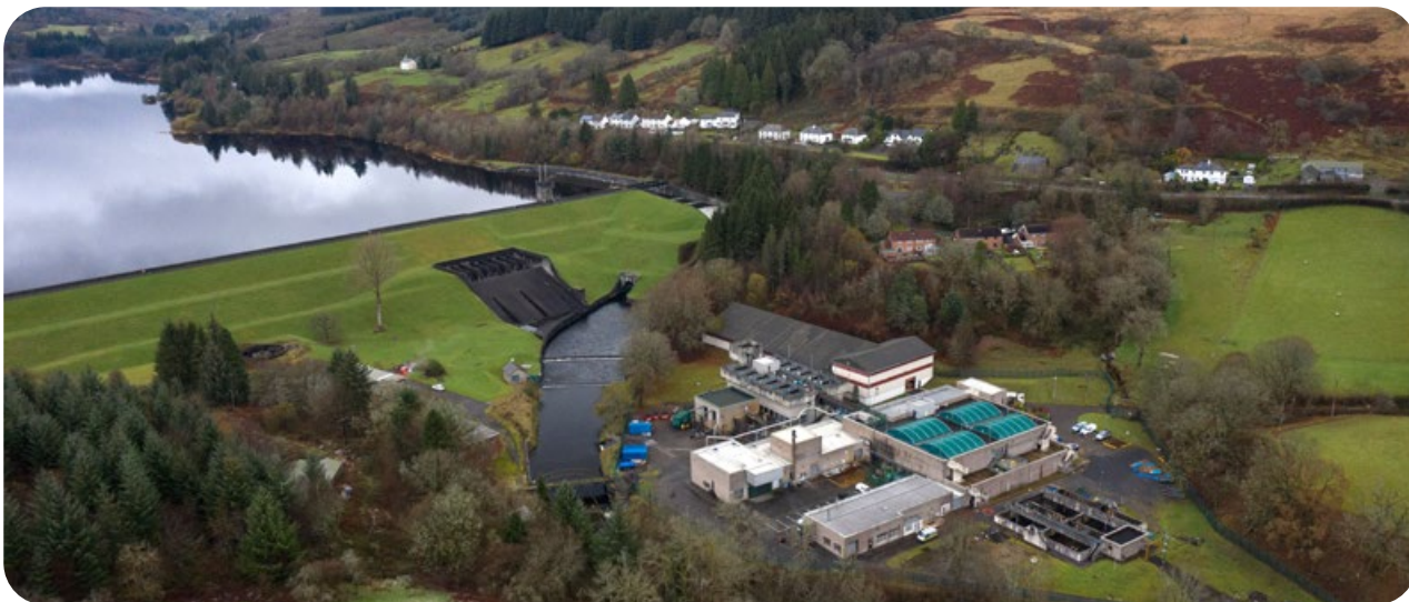
Llwyn-on water treatment works
