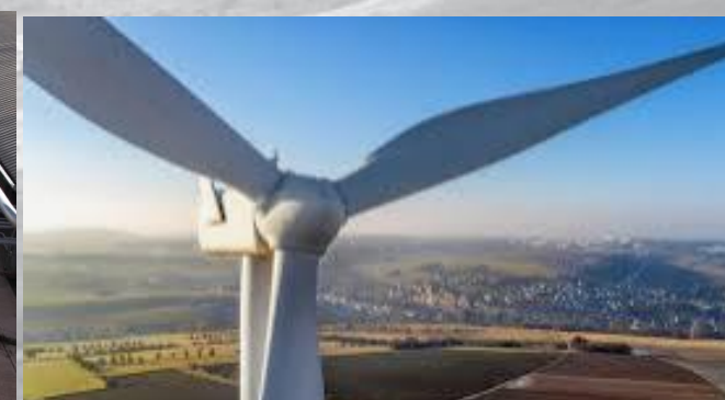
Wind turbines installed at both Nash & Swansea Wastewater Treatment Works
