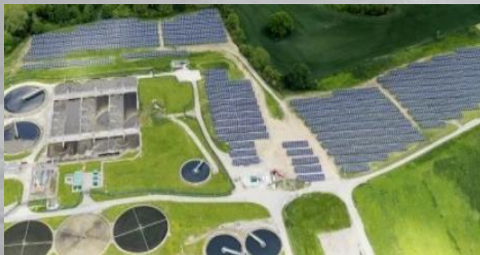
Five Fords Wastewater Treatment Works & Energy Park
