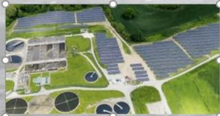
Five Fords Wastewater Treatment Works & Energy Park
