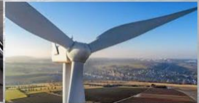
Wind turbines installed at both Nash & Swansea Wastewater Treatment Works
