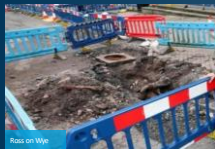
May Collapsed sewer
