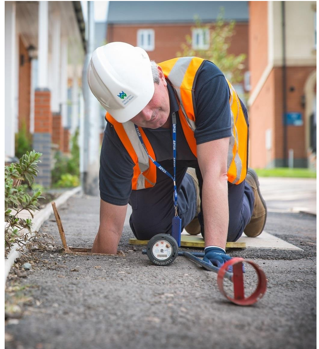
Figure 59 : Pipe replacement. © Welsh Water
