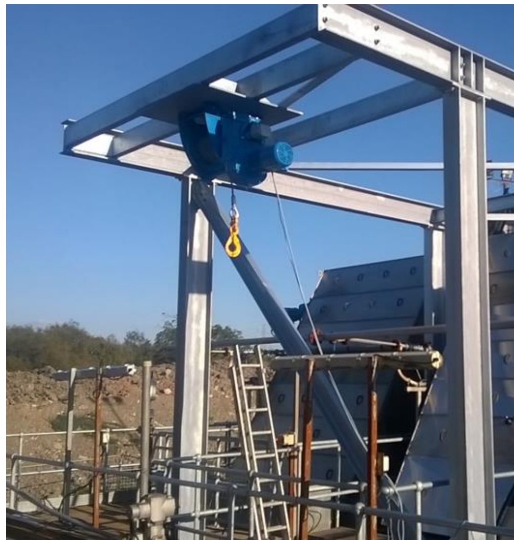
Figure 95: Newport Nash wastewater treatment works. © Welsh Water
