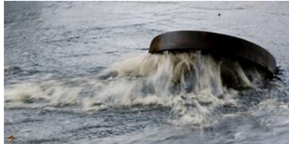
Figure 69 : Flooding on Carway Street. © Welsh Water
