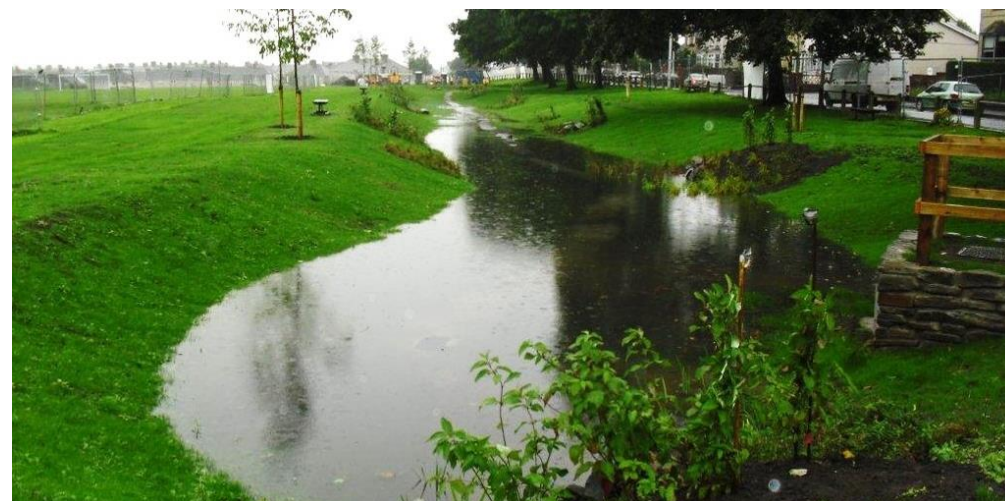
Figure 86 : A bioswale at Queen Mary's Walk, Llanelli. © Arup
