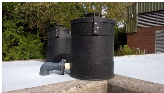
Figure 12: New glass reinforced plastic covers and passive filters at Barry West SPS (2016)
