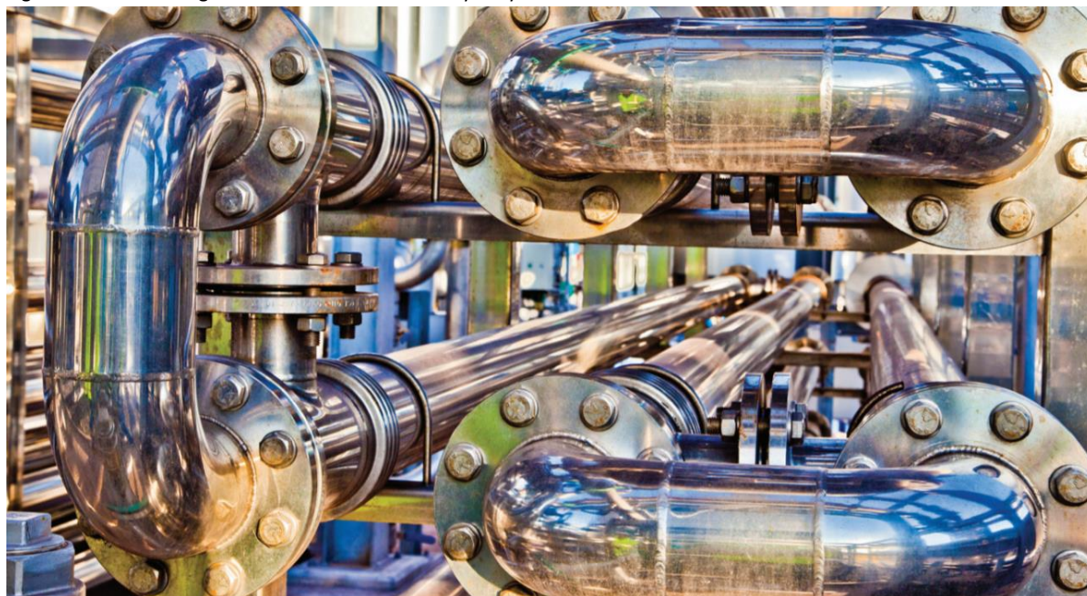
Figure 9: Heat Exchangers on one of Our Thermal Hydrolysis Plants
