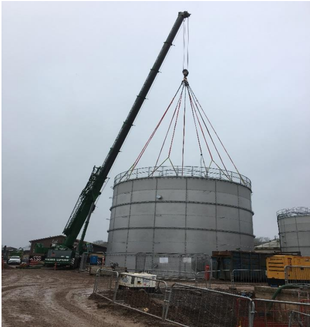
Digester being moved into place January 2020
