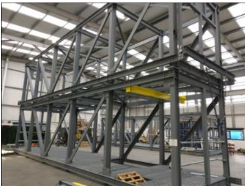
Boiler house being constructed offsite, Summer 2019
