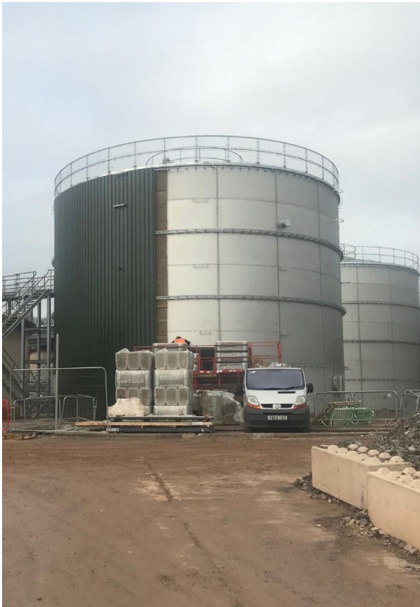
Digester being clad, March 2020
