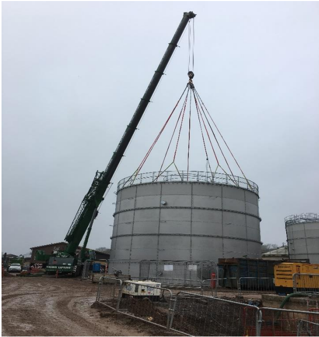
Digester being moved into place January 2020
