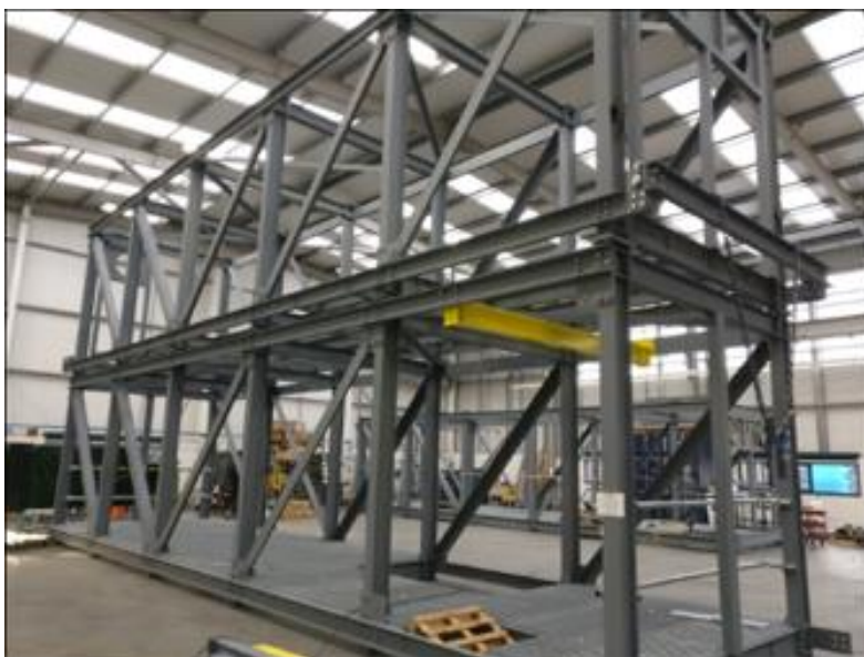
Boiler house being constructed offsite, Summer 2019
