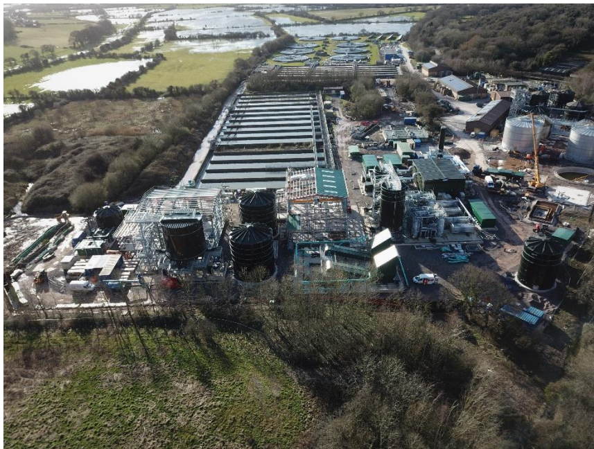
Cog Moors AAD under construction – additional digester installed onsite, March 2020
