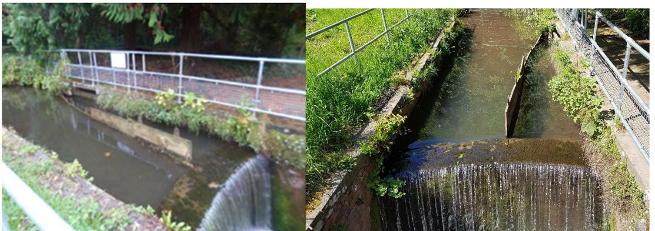
Figure 2-5 - Nant Fawr Intake Structure
