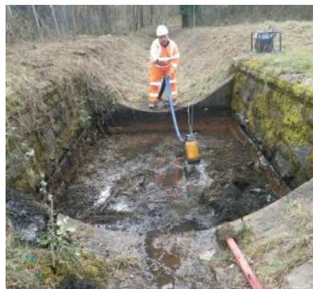
Photo: Specialist engineers clearing out one of the drainage chambers
