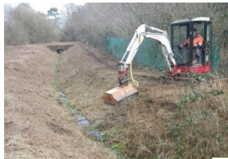
Photo: Specialist engineers clearing out one of the outflow channels
